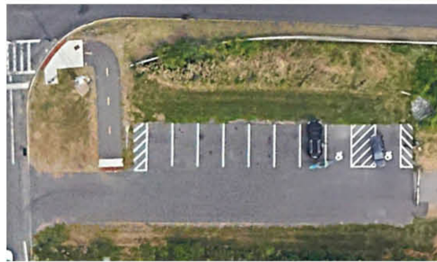
▲ Existing parking area
