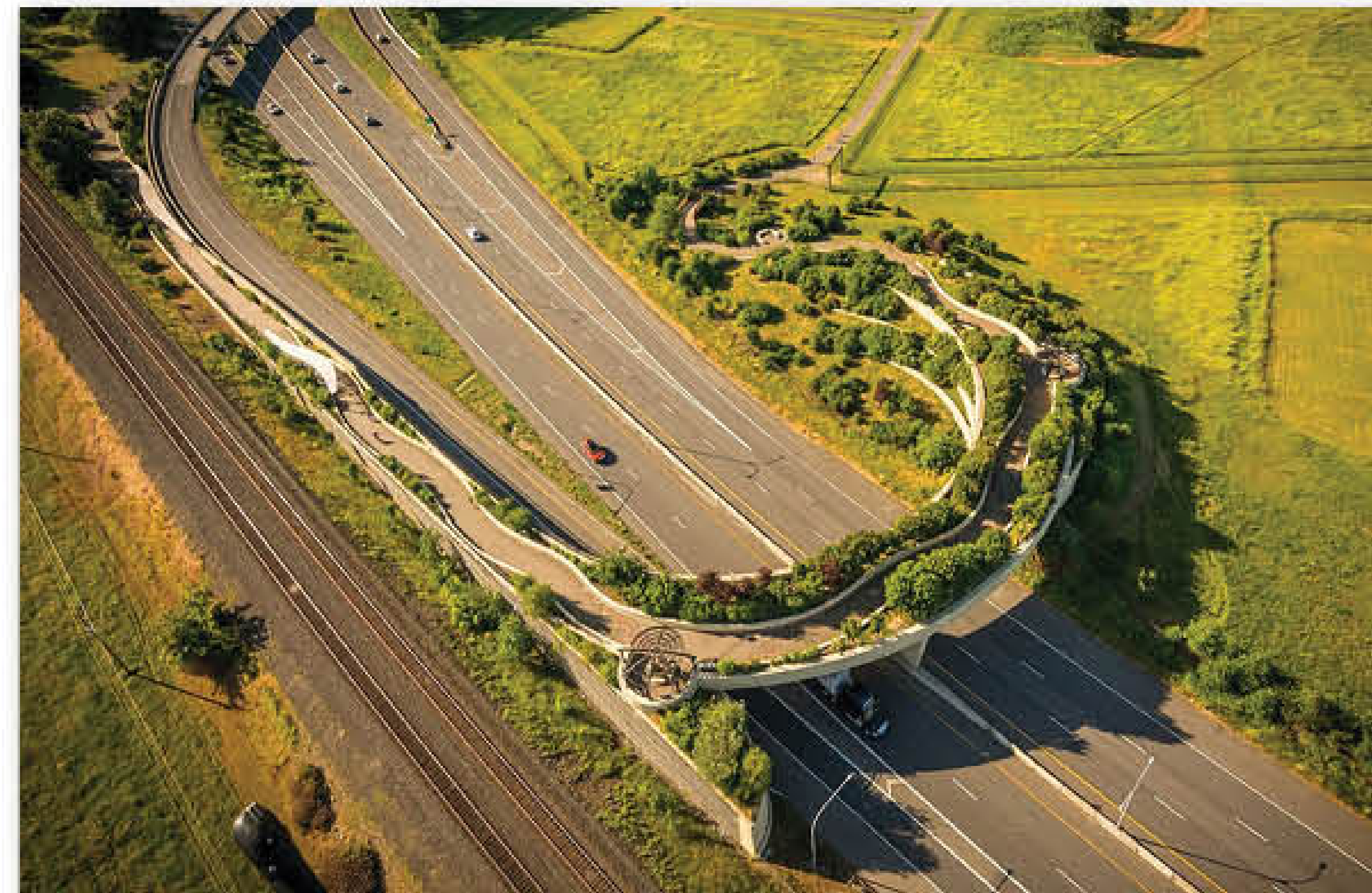
Vancouver Land Bridge, Vancouver, WA
