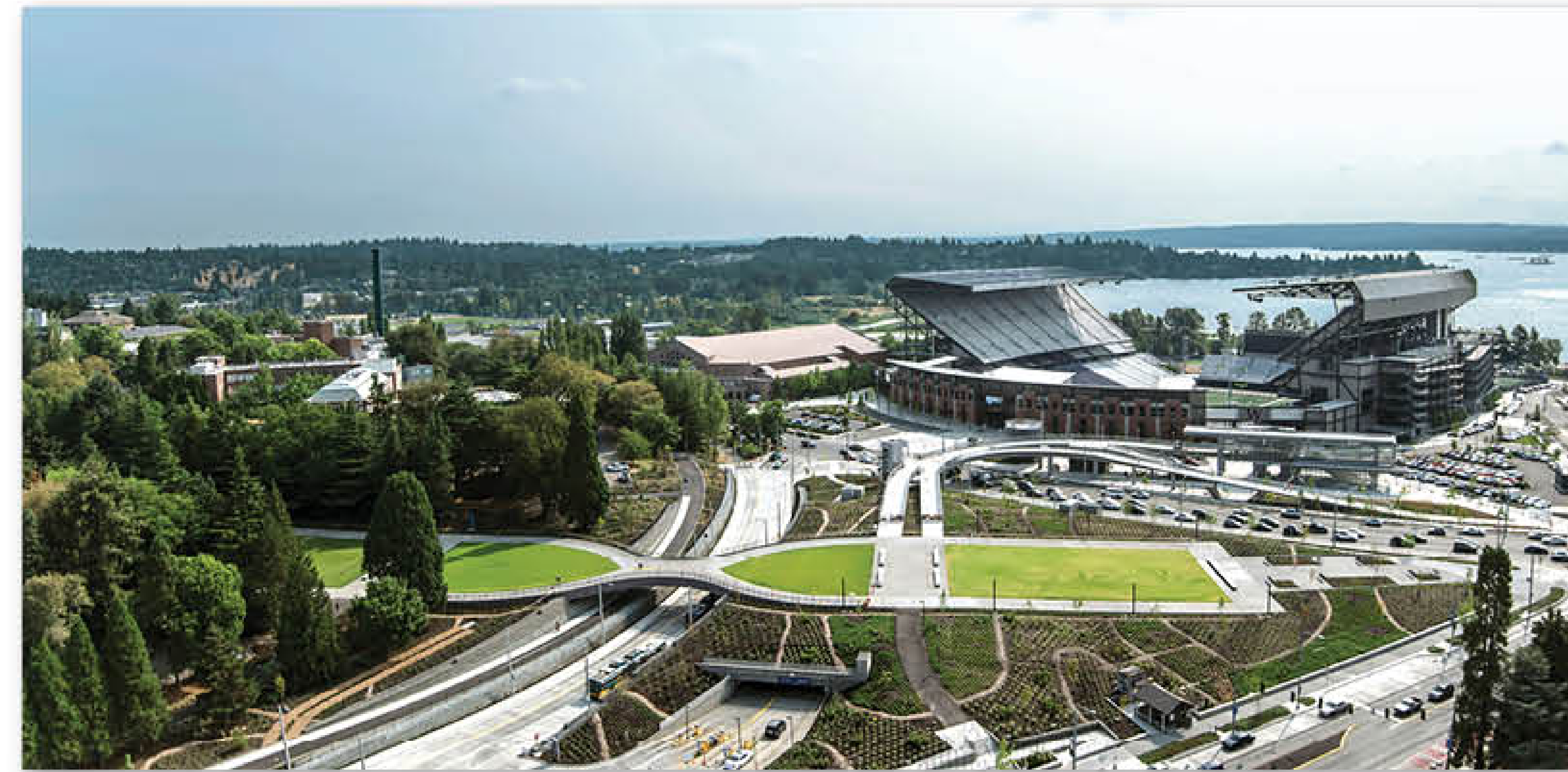
Lower Rainier Vista and Pedestrian Land Bridge, Seattle
