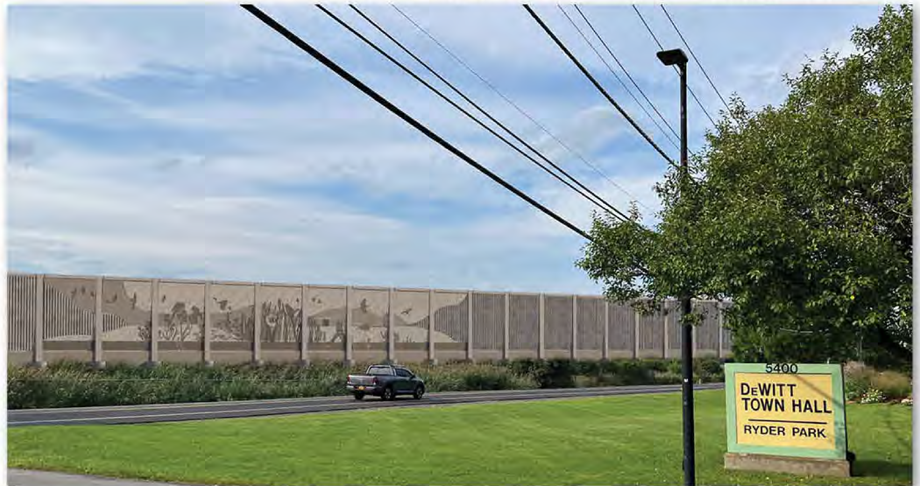
Future noise barrier 8B opposite DeWitt Town Hall ▼
