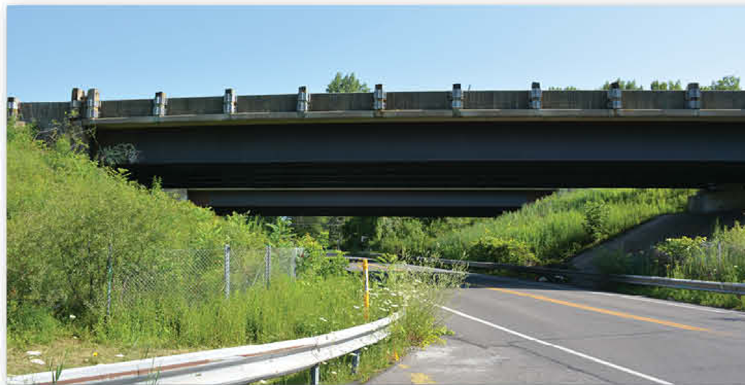
SB I-81 (existing I-481) over Totnam Road
