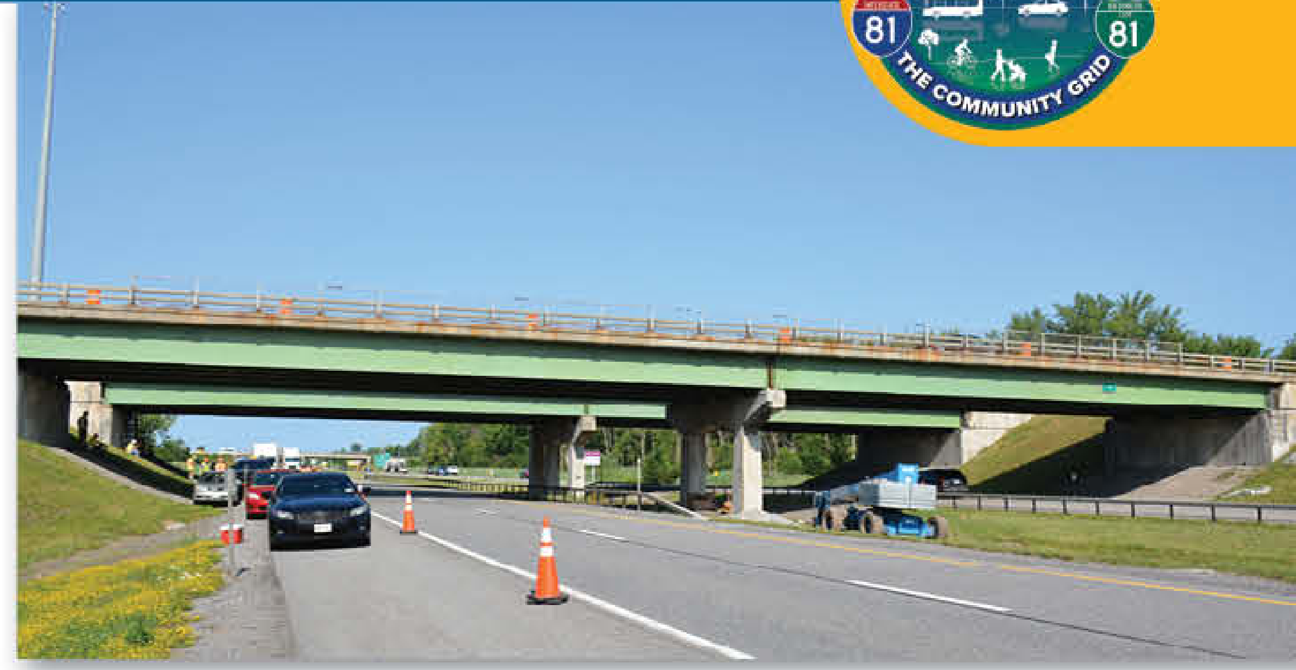
NB I-81 (existing I-481) over I-90 (NYS Thruway)
